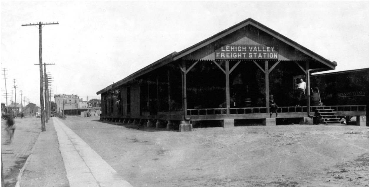
Perth Amboy, LV State St freight house June 7, 1912. RRSHS Collection
