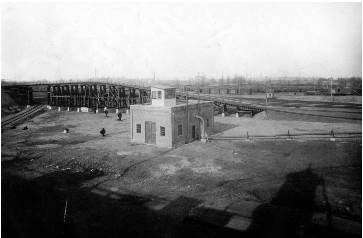
Perth Amboy, 1916, LVRR coal pier cable house, looking generally west. RRSHS Collection
