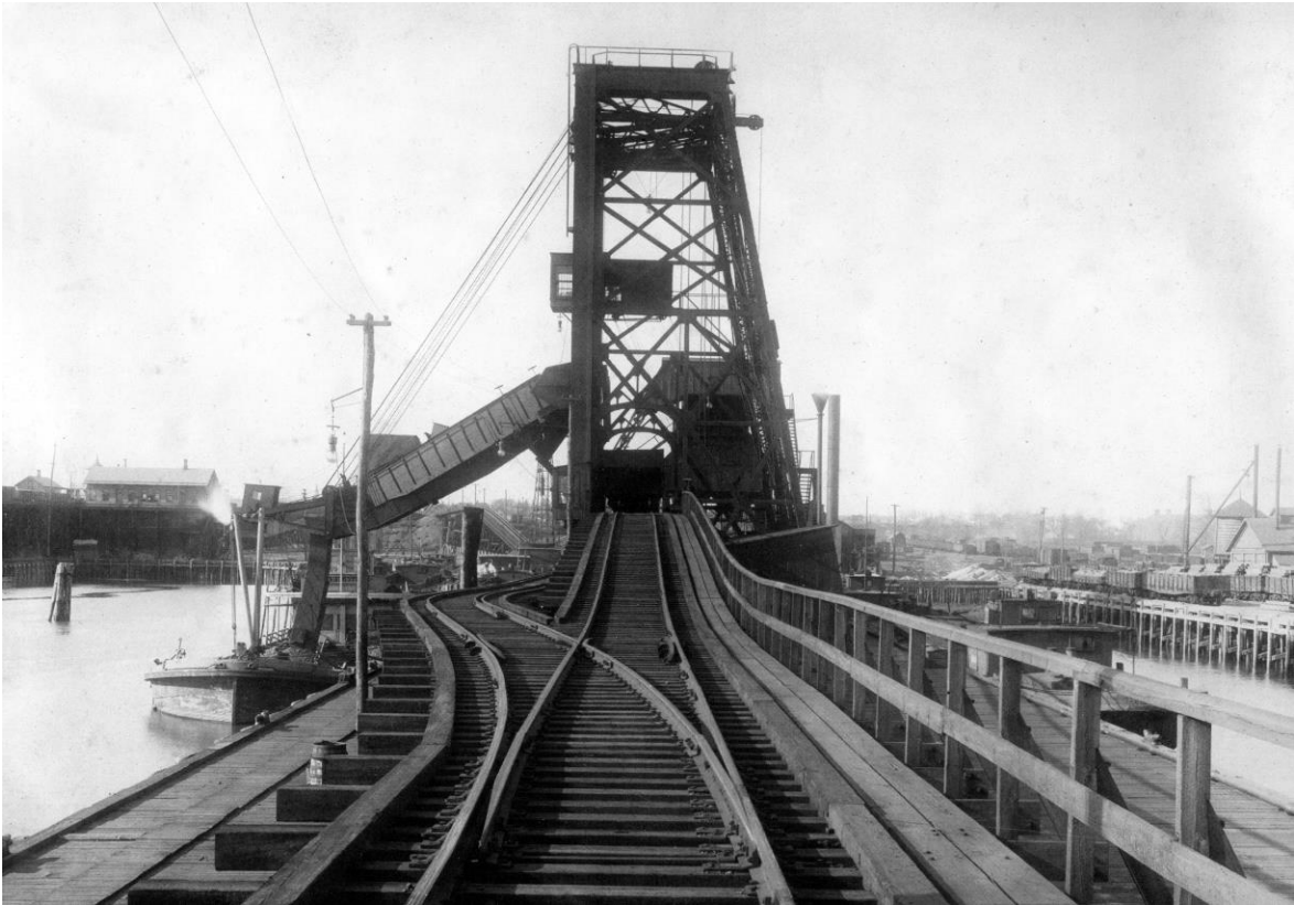
Perth Amboy, LVRR Pier C McMyler coal dumper circa 1916. RRSHS Collection
