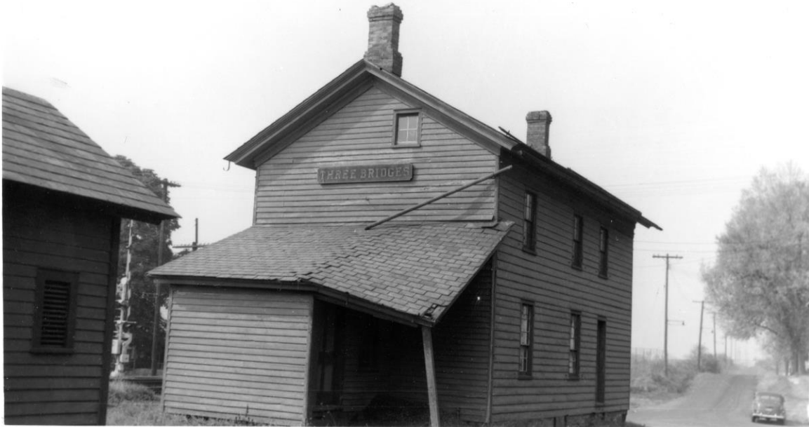
Three Bridges, rear and side view, it looks like the B&B gang has not done much maintenance here recently! August 23, 1956 RRSHS Collection
