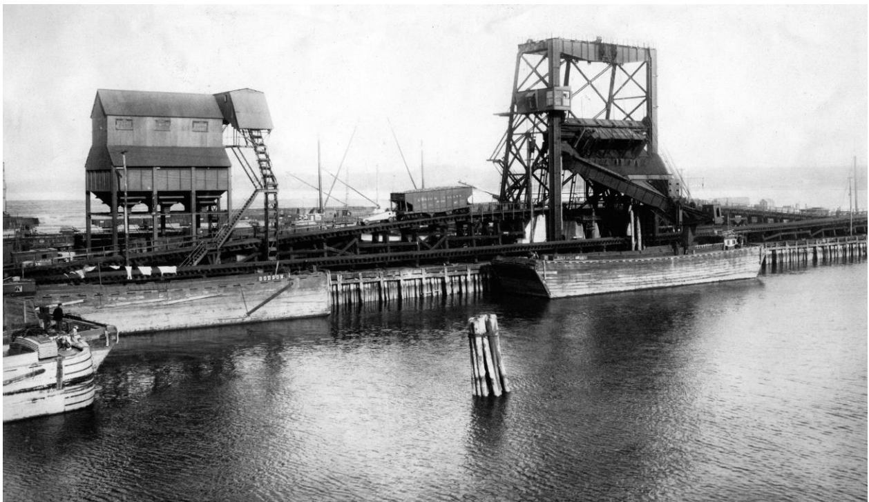
Perth Amboy's Pier C, circa.1916 with barge unloader (left) and McMylor coal dumper (right). RRSHS Collection.
