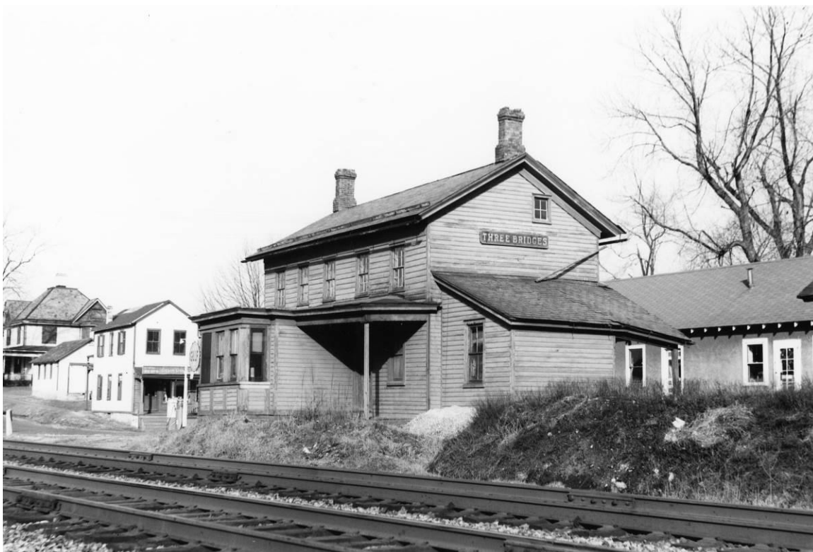
Three Bridges architecturally resembled a rural home. December 21, 1953, Ed Weber photo. RRSHS Collection
