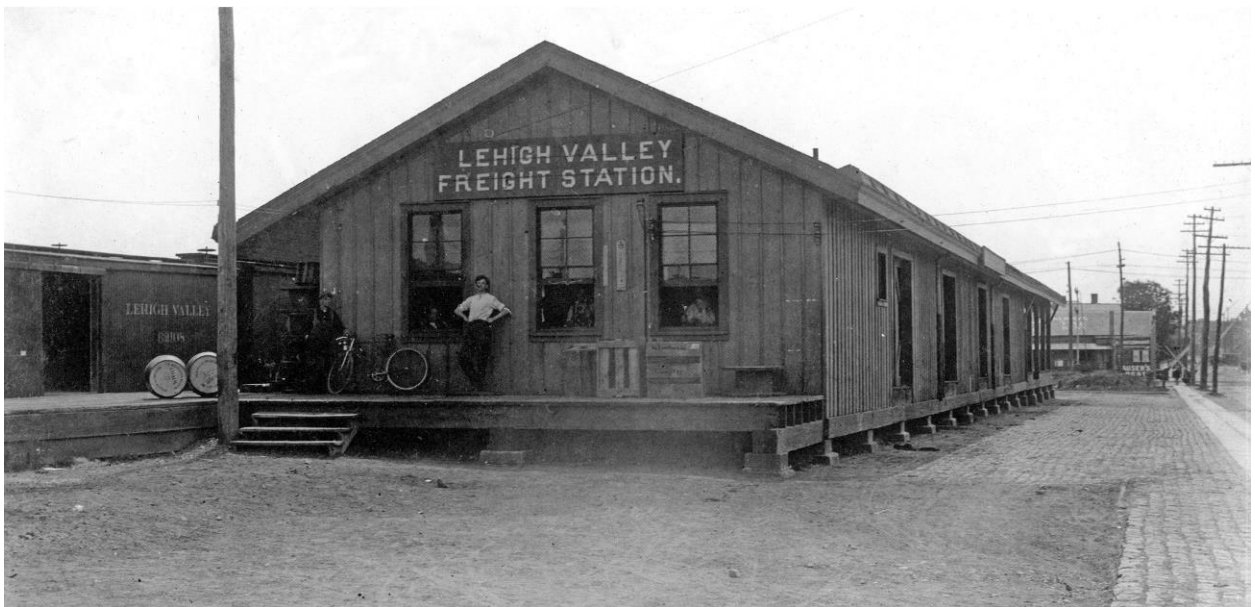
Perth Amboy, LV State St freight house June 7, 1912. RRSHS Collection
