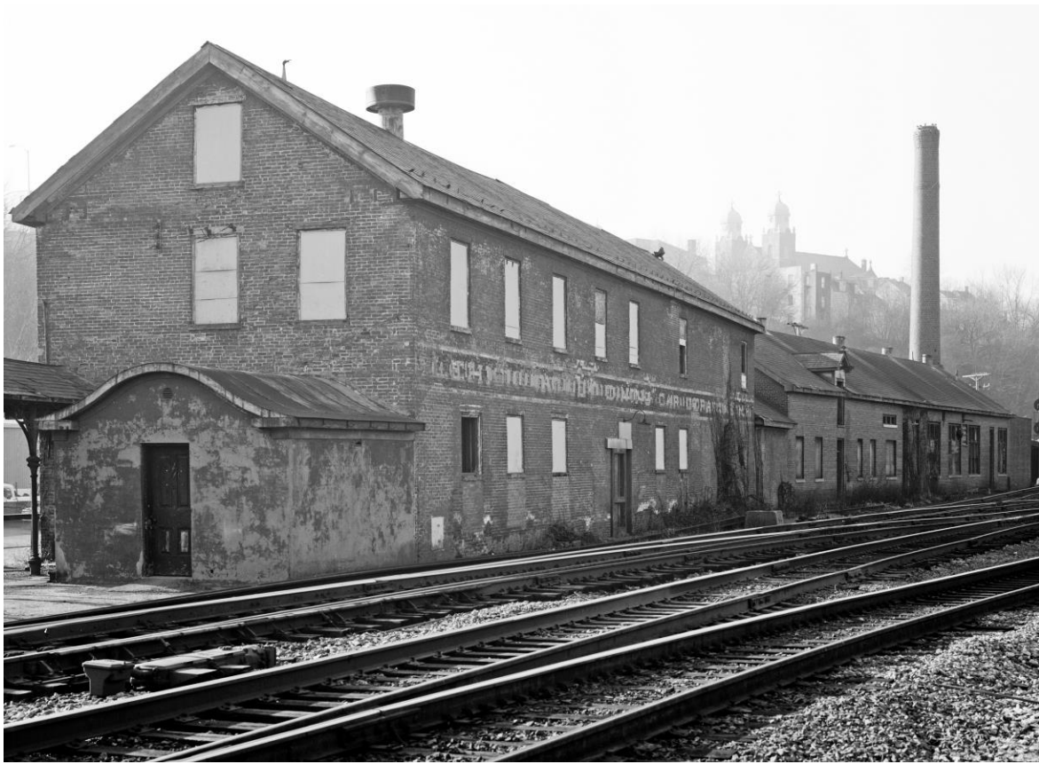
Easton, PA LV dining car department commissary. The building dates to 1868 and originally served as the second LV station in Easton. Undated photo, RRSHS Collection.
