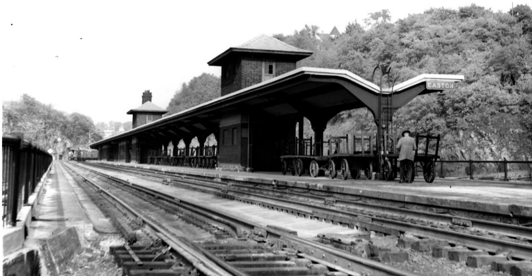
Easton, PA, LV passenger station platforms. Opened February 27, 1927, this was the final LV depot for Easton. Of a unique design, track and platforms were above the baggage and express handling portions of the facility. Undated photo, circa 1953, by Ed Weber. RRSHS Collection.
