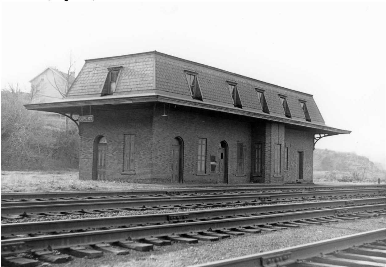
Coplay, PA LV station dated to the 1880s, Architecturally unique, it featured a slate Mansard roof. November 16, 1952. Ed Weber, RRSHS Collection
