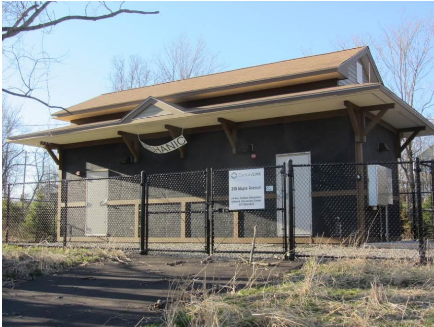
NESHANIC STATION (MP 44.7) Although not actually a station, this structure gets “honorable mention” for looking like a station, and is located on the same site as the former station. It was constructed in 2017 by Century Link, a fiber-optics company, and functions as a “fiber-node” where fiber-optic signals are amplified and branched out to other lines. April 10, 2019
