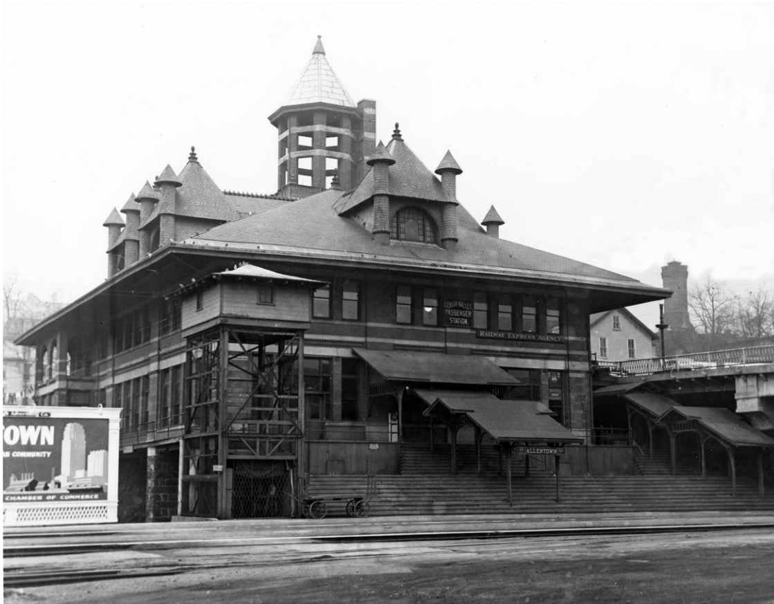
Allentown, PA. The LV station was constructed in 1890 over Jordan Creek on piers. The top floor was level with Hamilton Street. The track canopies have been removed, and we are looking west. November 24, 1950 Ed Weber, RRSBS Collection
