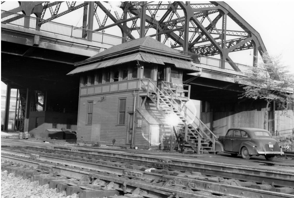
Bethlehem, PA May 9, 1953 LV-Reading interlocking tower, milepost 88.6, built 1928. Ed Weber photo. RRSHS Collection (Ed. Note: photo has some damage in the center.)
