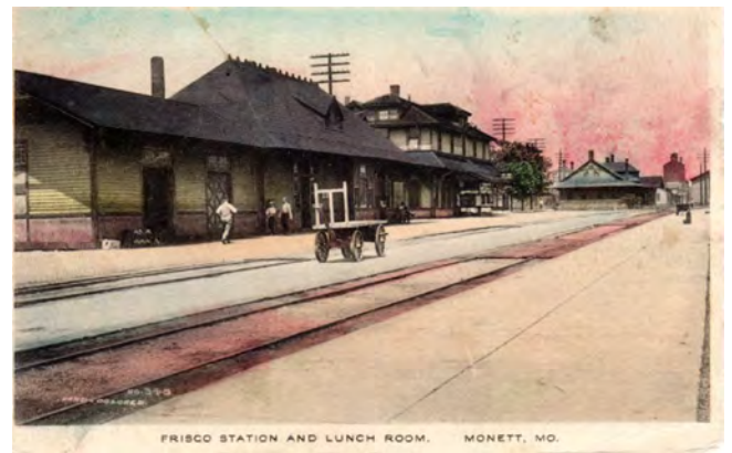
MONETT, MO Frisco: The one story station is on the left with the lunch room the two story building in the middle of this hand colored postcard. It has an RPO cancel from train No. 4 dated sometime in 1911. One wonders if the third building may be a hotel for employees. During the period of Santa Fe control, the Fred Harvey built two story eating houses with the Harvey girls staying on the second floor. By 1911, the Harvey chain had abandoned the Frisco locations. Kent Hannah collection.
