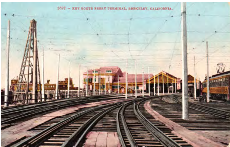
BEREKLEY, CA Key Route Ferry Terminal: The train shed is to the right side of the transfer building on the mole. Stored cars are in the yard on the extreme right. There is a double ended ferry on the left side of the mole terminal. The card is dated March 1910. Kent Hannah collection.
