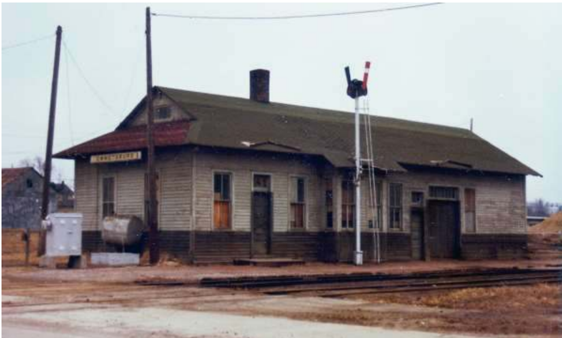
April 8, 1979 Spencer Note the two sets of train order boards: The top is set was for the “mainline” that ran from Mason City to Mitchell SD; the bottom set is set for the “branchline” that ran from Sprite Lake (from the north) connecting with the mainline west of the depot to Rockwell City (from the south) connecting with the mainline east of the depot.
