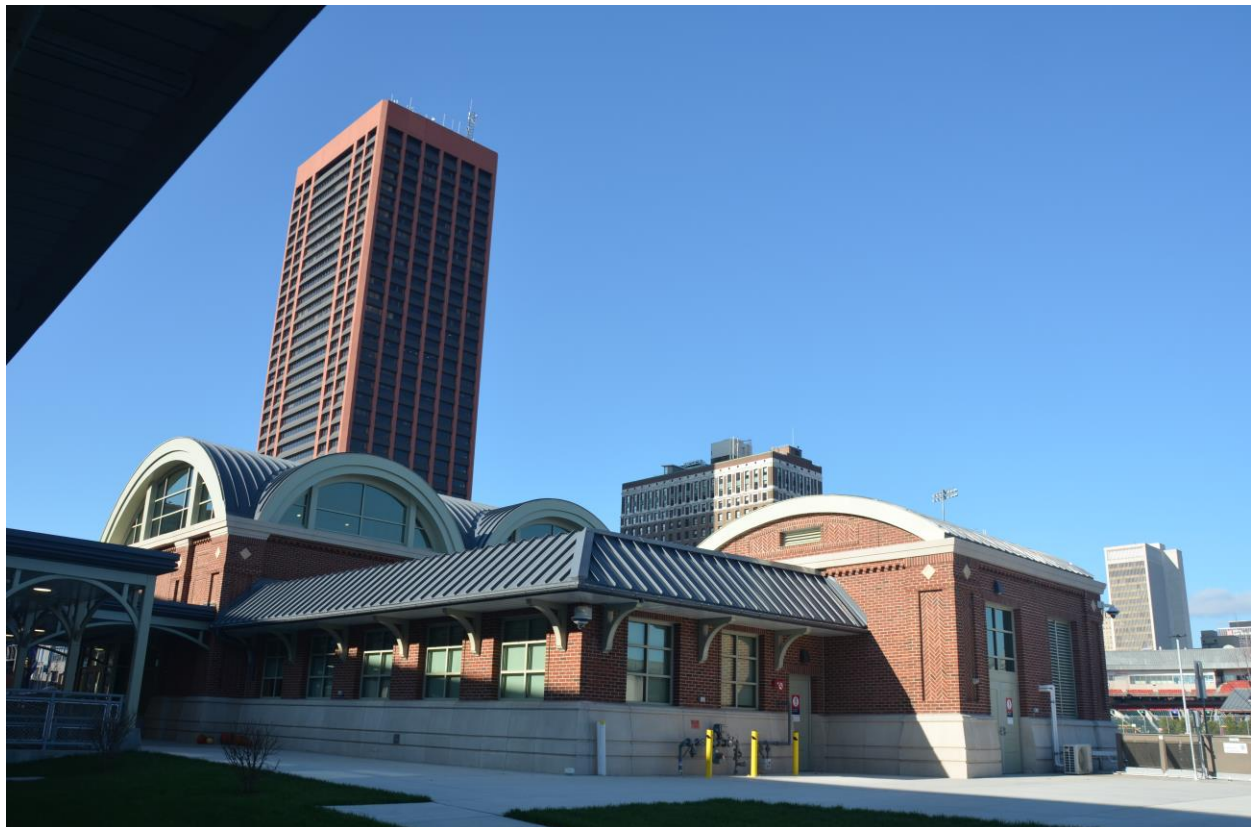
Trackside view of the station. Its location is nearly beneath Interstate 190 highway overpasses. In the background is the Seneca One tower, at 38 stories, Buffalo's tallest building. All photos, November 14, 2020, John C. Dahl.
