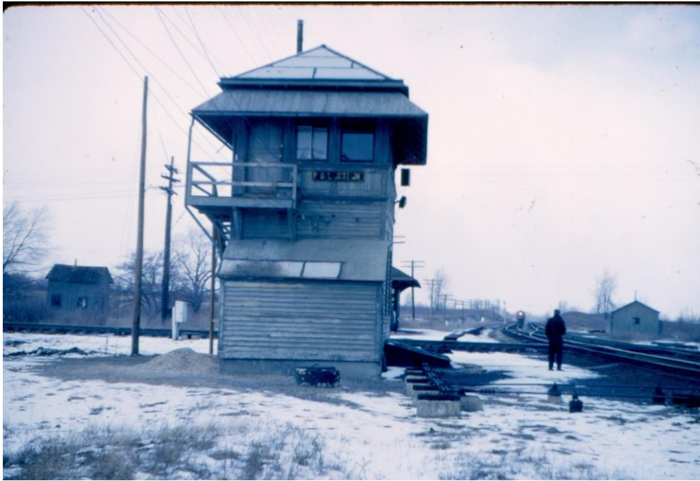
P&L Junction, NY – The interlocking tower of typical LVRR design was opposite the depot, a corner of which can be seen just to the right of the tower. It is March 19, 1965 as the towerman waits for an approaching train to hand up orders. Brian Angevine collection.
