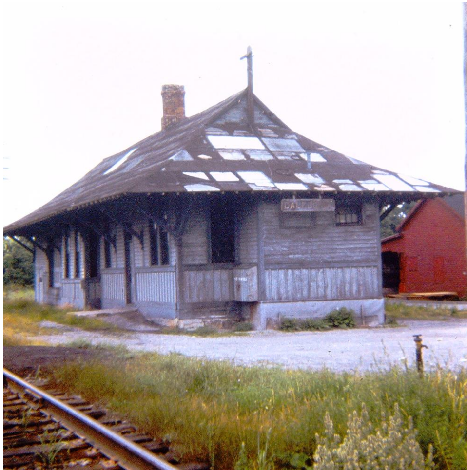
Caledonia, NY - In a snapshot view, on July 18, 1971 the depot is still intact, probably in use by the railroads signal maintainers or bridge & building gang, if the Lehigh had much of any such staff left by that point in time. Someone is obviously patching the roof in a battle to arrest the onslaught of deterioration and time. Paul Templeton collection, courtesy Jeff Kovacs.
