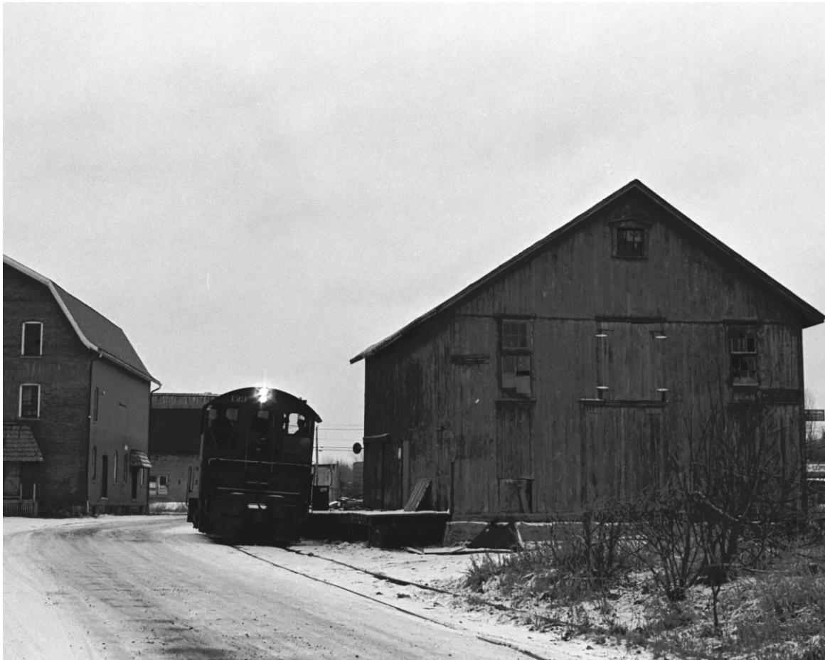
Victor, NY – was this possibly the freight station located on a spur line, with what is identified as train RM-2? The structure is said to have been lost in a controlled burn in 1990. Jeff Kovacs collection.
