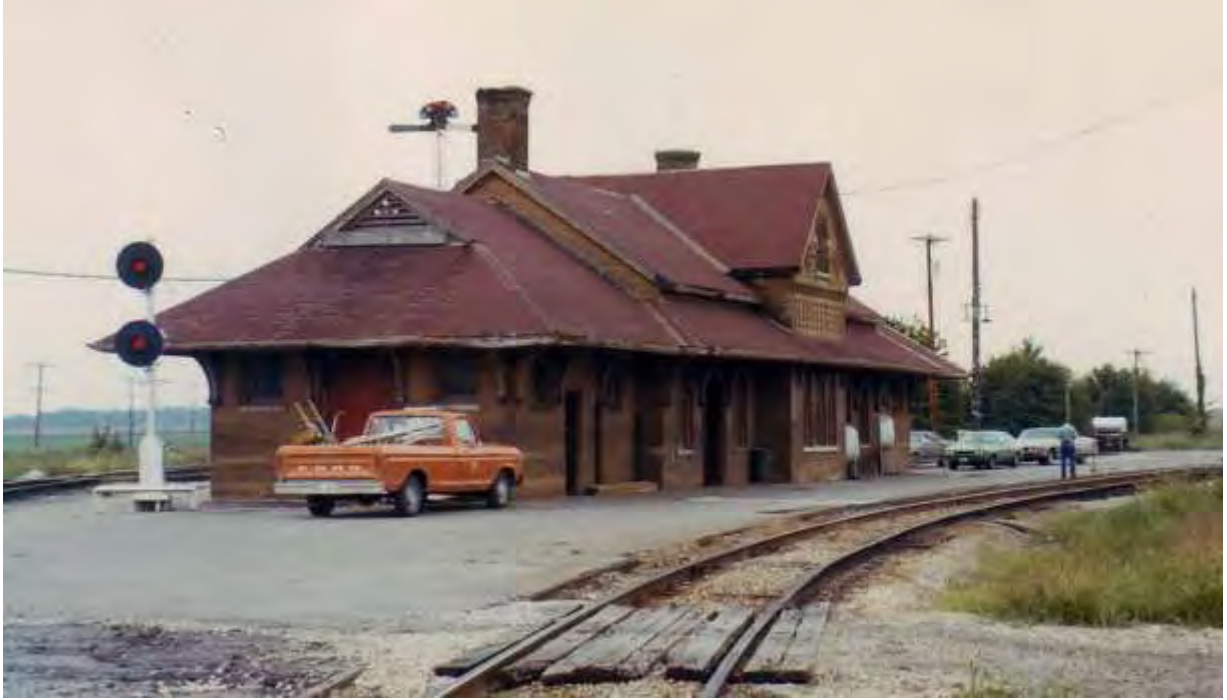
West Liberty on August 5, 1977 Junction of two RI lines, view of the “back” of the depot on the connecting track, diamonds on front side of depot.
