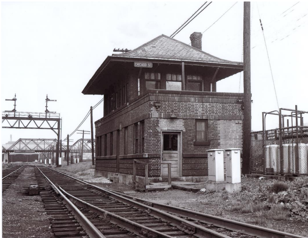
Buffalo, NY – near the throat of LV's downtown passenger station and adjacent express handling stood the modern Chicago Street tower. Brian Angevine collection
