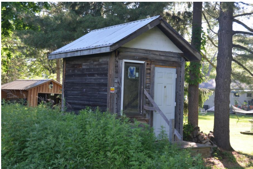
Tonawanda Junction – After the two level tower was removed about 1920, a set of crossovers on the joint NYC-LV trackage was controlled by levers in this ground interlocking a few hundred feet west of where the tower had been. The switch to the old NYC Peanut was just behind this photo's camera position. Remarkably, the switch shanty still stands in its original location, although all track has long been removed. It now functions as a garden shed. A few telegraph poles still hold on nearby as well. June 24, 2022 photo, John C. Dahl.
