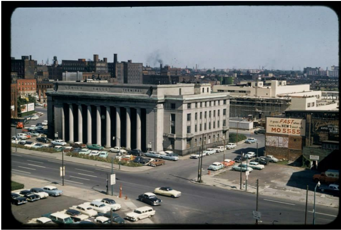
Buffalo, NY – The train concourse and shed have already been demolished in this late 1950's view with new construction on the site in progress. The head house building's days are numbered before it too will sadly fall to the wreckers. Private collection.
