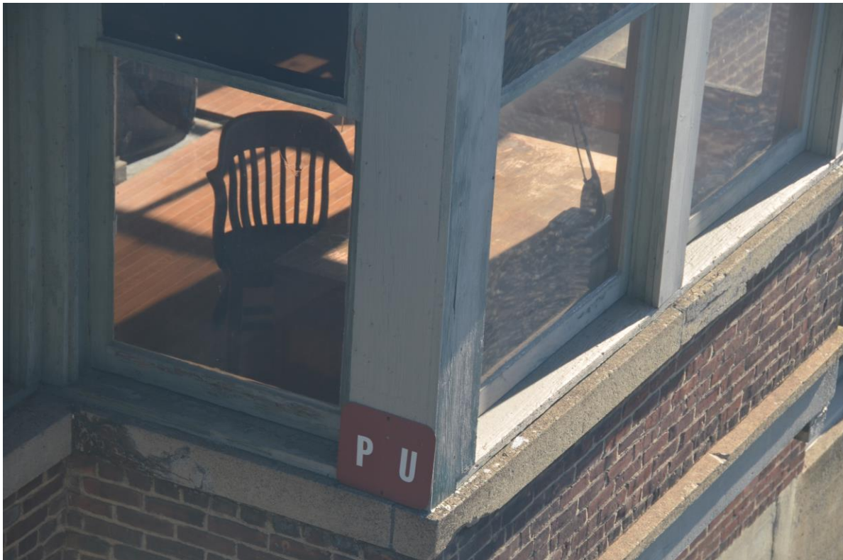
Philipsburg, NJ – the operator’s chair has been vacant since the last controlled movement thru ‘PU’ when New Jersey Transit ended commuter service to the city in 1983. In 2007 the tower was acquired by Ron and Jeane Titus and has been undergoing restoration as a landmark. August 18, 2022.
