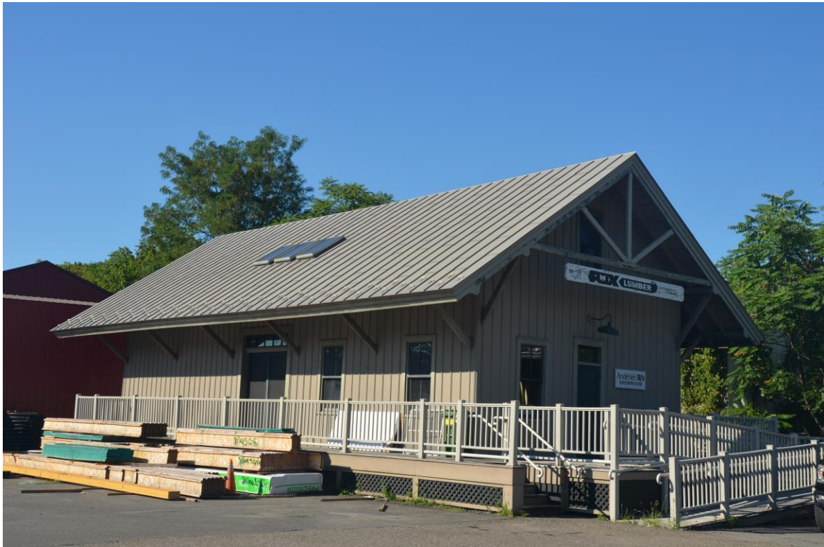
Clinton, NJ – Lehigh Valley built this freight station and a passenger depot at the end of the 1.8 mile Clinton branch. August 18, 2022
