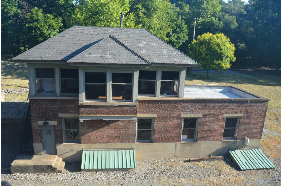
Philipsburg, NJ – “PU” tower of the Central RR of New Jersey opened in October 1921. A modern interlocking, it served during some of the CNJ’s best years. The former DL&W ‘Old Road’ tracks are located just beyond the trees behind the tower.
