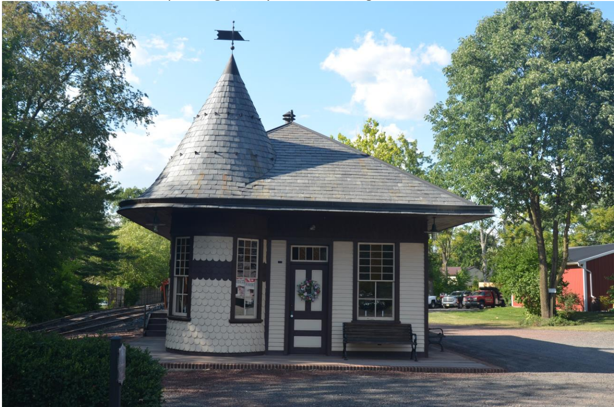
Wycomb, PA – The Reading Railroad is known for its Victorian era classic stations, and this circa 1890 station is well maintained by the tourist train line. August 18, 2022.
