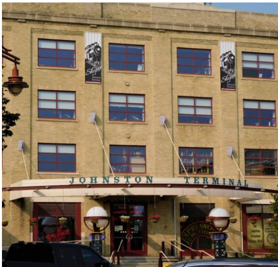
Winnipeg, Manitoba - Johnson Terminal Building, The Forks
