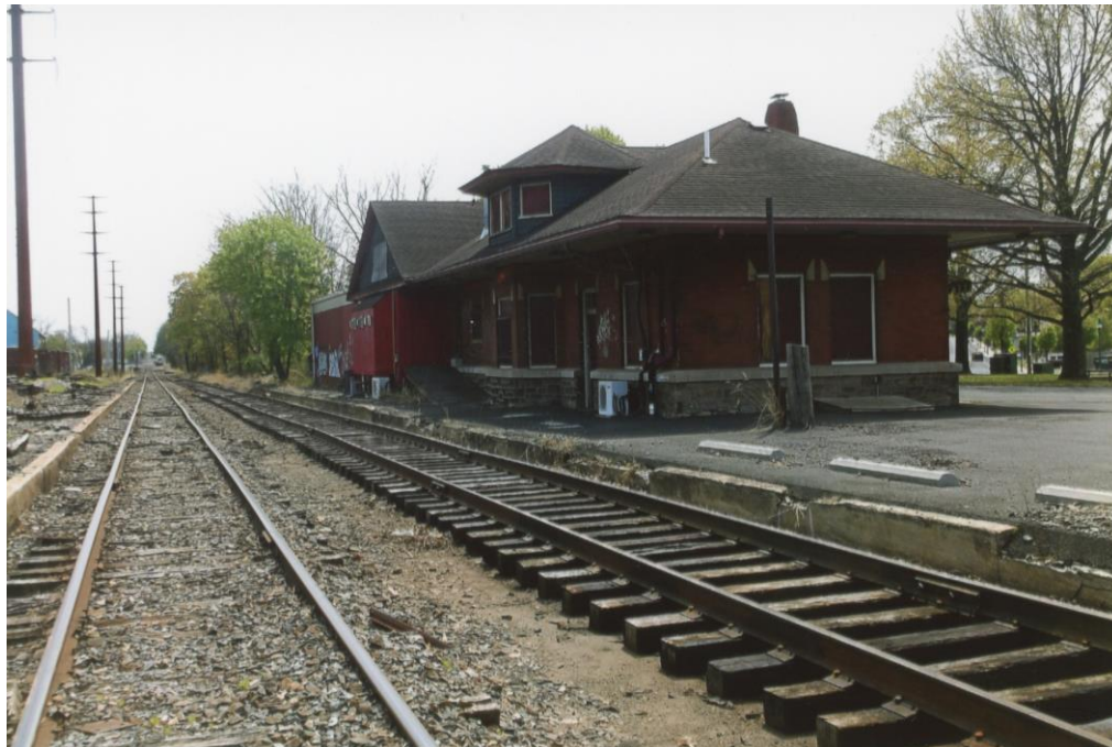
Hatfield, PA – Reading RR. This view looks towards Philadelphia. The south end of the structure has been modified with an addition. April 2022.
