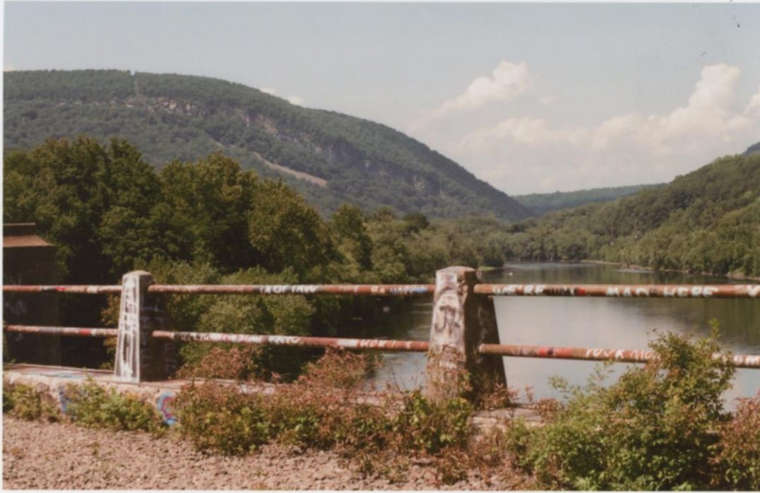
8.13.21 ON DELAWARE VIADUCT LOOKING UPSTREAM
