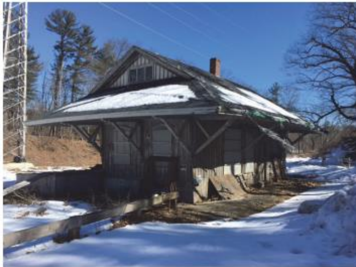
The Weston Combination Depot features a standard gabled-hip roof, similar to the station surviving in Wayland. In 1912 the station was moved about 200 feet east as part of a grade crossing elimination project. (Photo by Rick Conard, March 2021. Caption info from A Field Guide to Southern New England Railroad Depots and Freight Houses by John H. Roy, Jr.)
