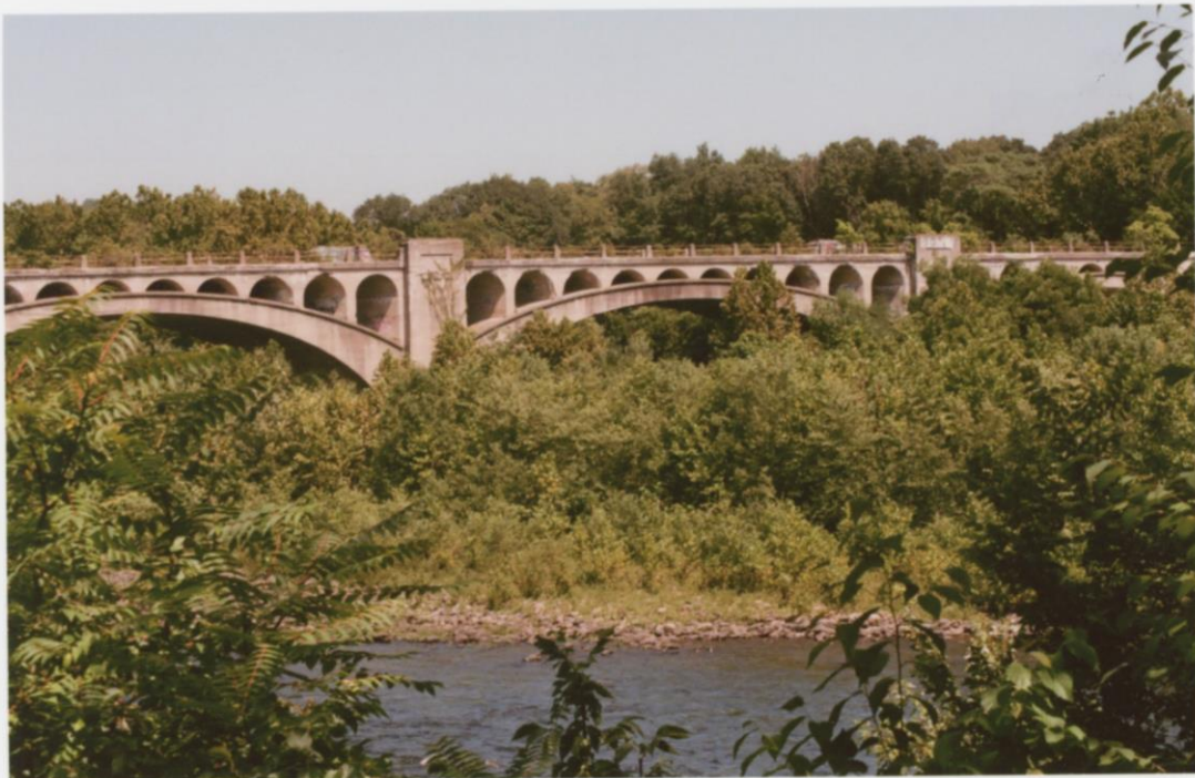
8.13.21 DELAWARE VIADUCT COLUMBIA N.J. SIDE 1300' LONG 1912
