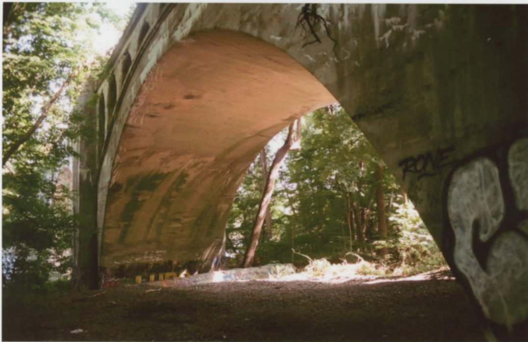
8.13.21 PA. END DELAWARE VIADUCT
